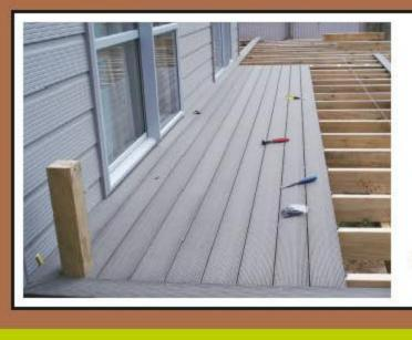
Accessories 1 clip & screw required on each joist
